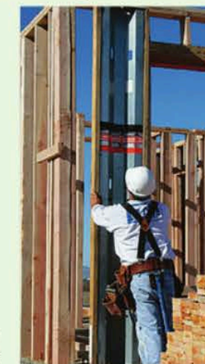
Strong Identity. Simpson Strong-Tie offers a range of products for strengthening connections and walls, including the Strong-Wall Shearwalls pictured here. www.strongtie.com
