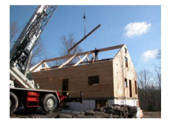
Enertia® homes are clear-span, or with just a few load-path posts - which means the interior partitions are not load bearing and can be placed freely.
